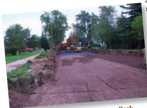
Preparing for paving in Billings Park
