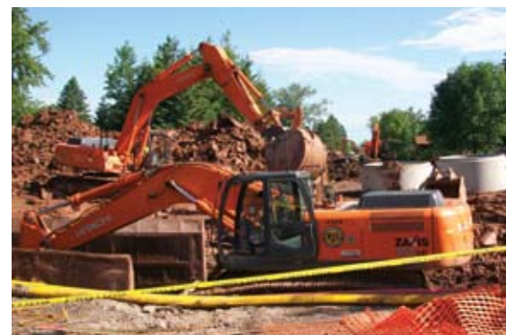
South Superior storm sewer work
